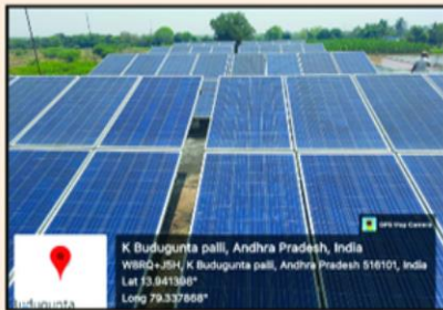
Solar Power Facility
